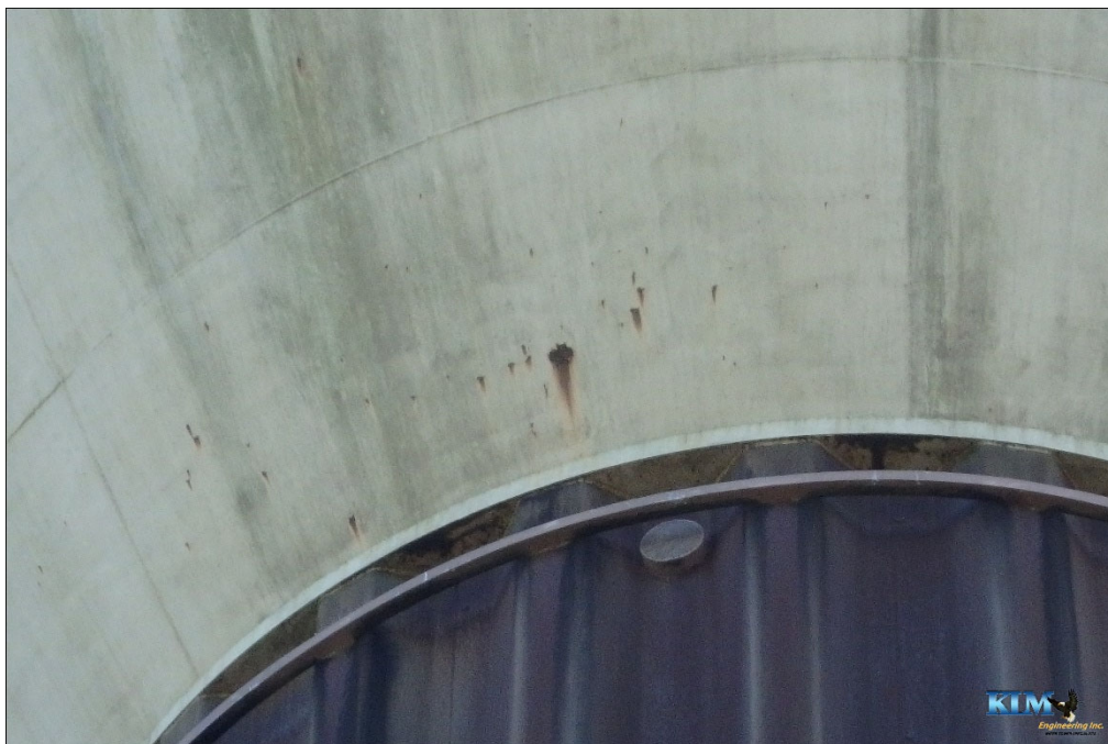
Photo No. 58 Condition of exterior coating near base of tank Spot and surface corrosion visible
