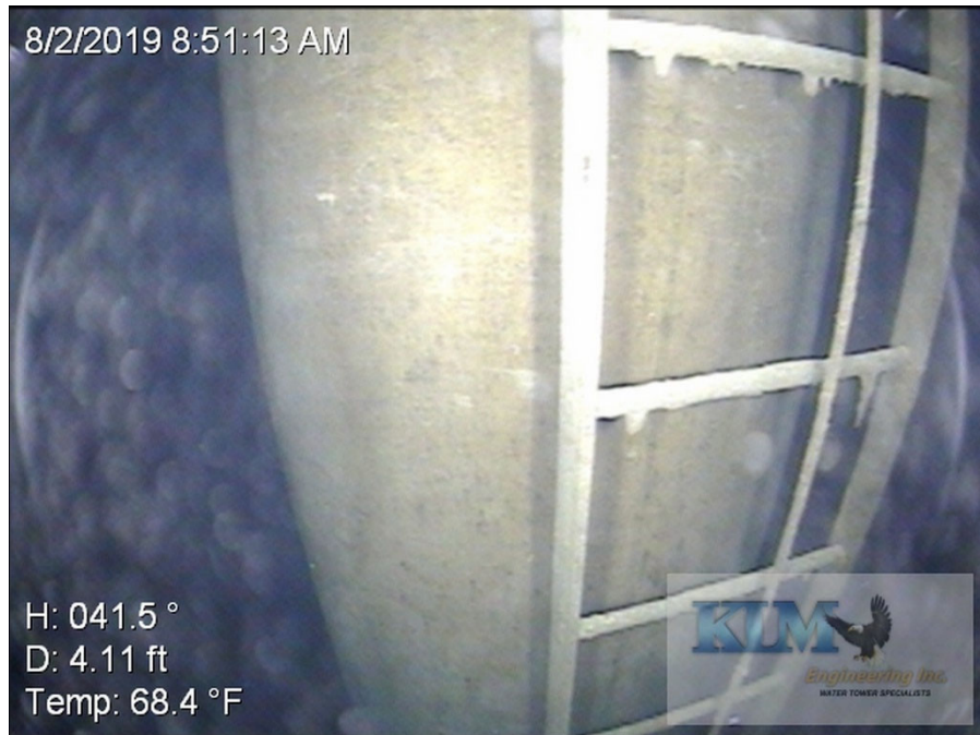
Photo No. 7 Condition of interior wet coating on drywell tube below HWL
