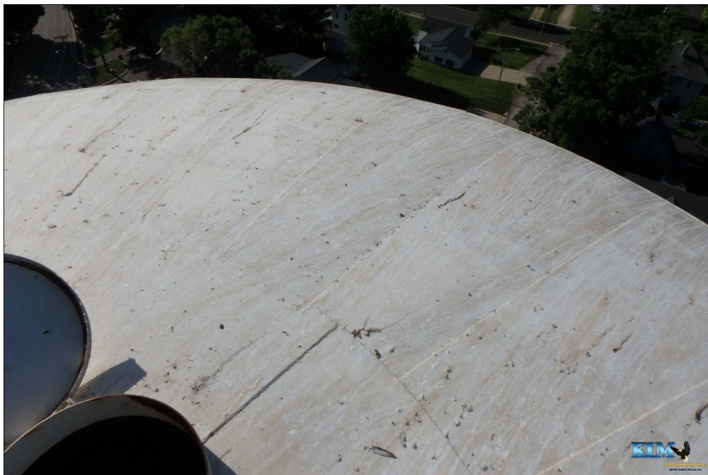
Photo No. 56 Condition of exterior coating on roof Bird droppings covering roof
