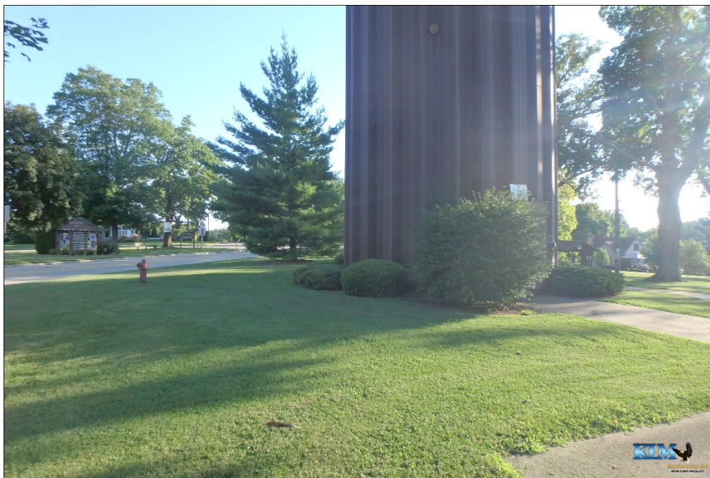
Photo No. 64 Site conditions near base of tower Hydrant for maintenance needs visible
