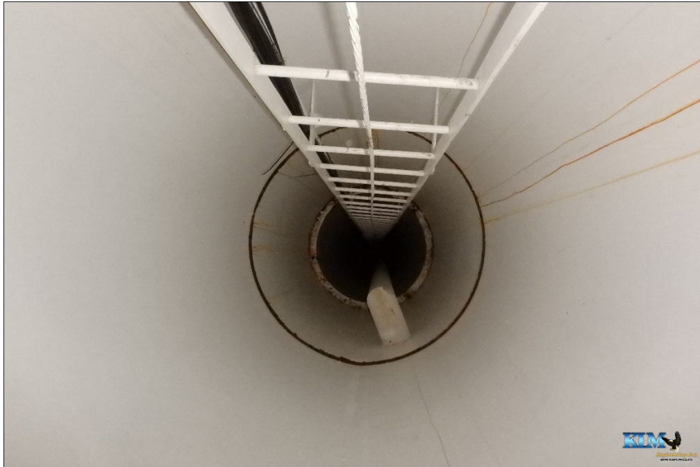
Photo No. 23 Condition of interior dry coating inside drywell tube; view looking down tube
