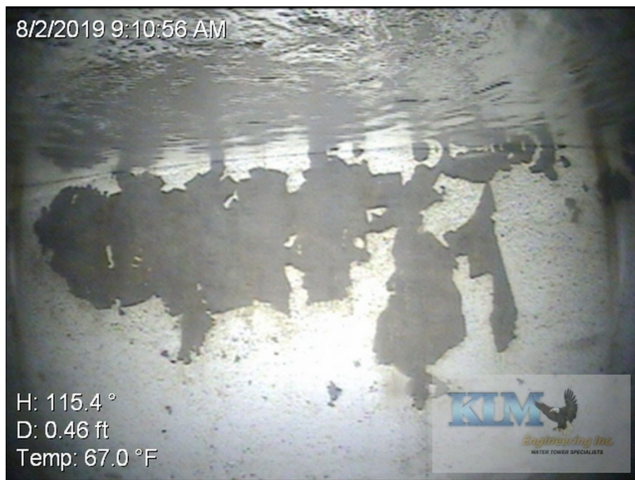
Photo No. 10 Condition of interior wet coating just below HWL Dark scale formation on shell
