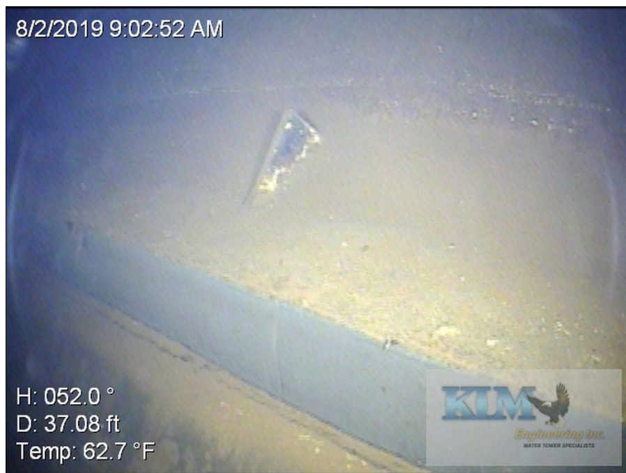
Photo No. 16 Condition of interior wet coating near tension ring Heavy sediment accumulation visible
