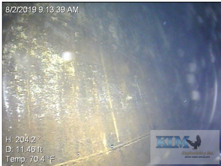
Photo No. 13 Condition of interior wet coating on shell wall Heavy staining and scale development
