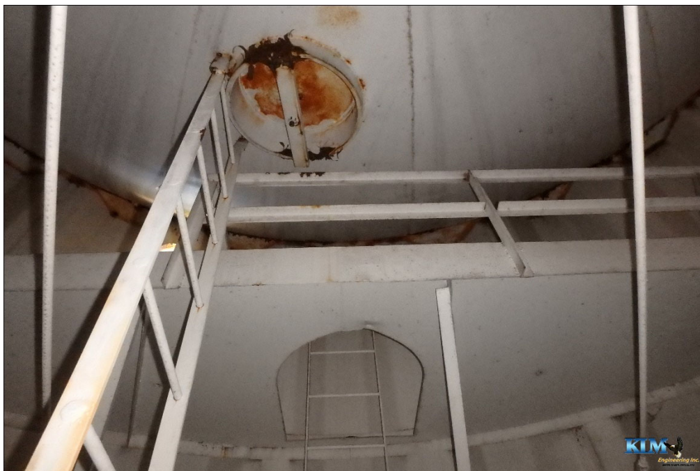
Photo No. 31 Condition of interior dry coating on bowl at bowl manway Random locations of heavy coating peeling and surface corrosion
