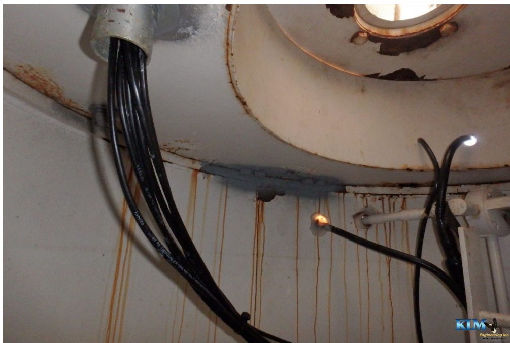
Photo No. 21 Condition of interior dry coating at top of drywell tube Significant peeling and surface corrosion occurring
