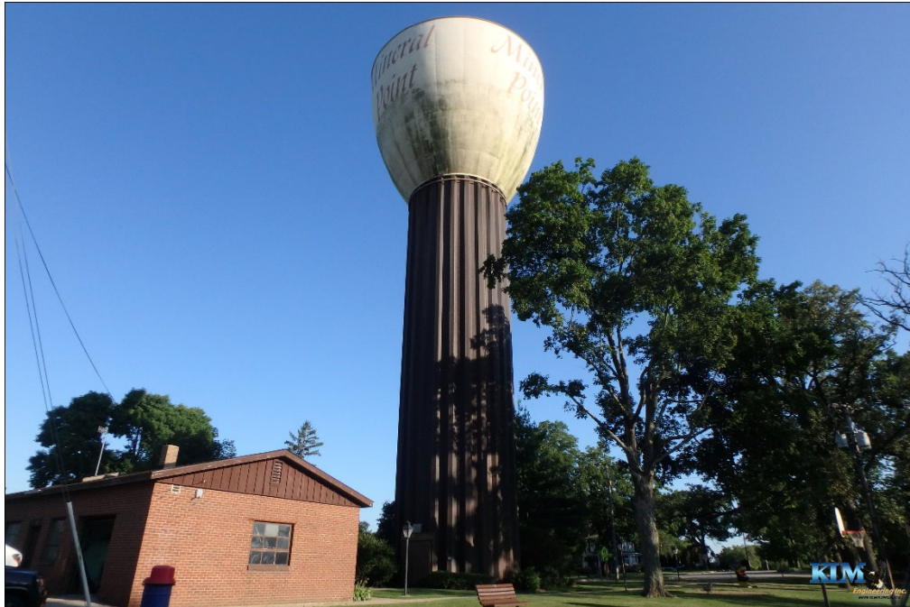
Photo No. 1 Overall view of tower
