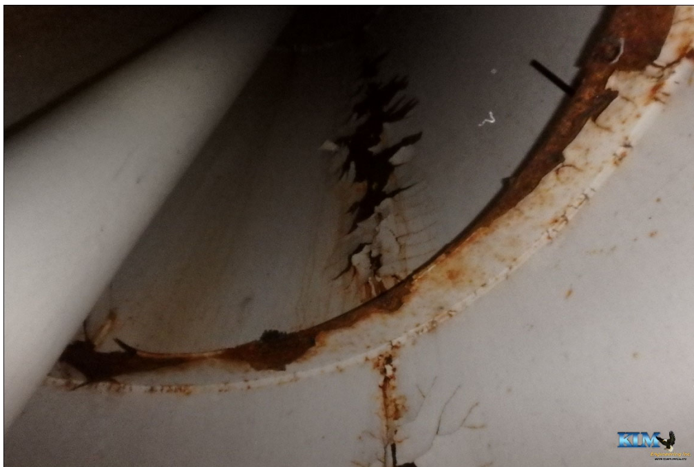
Photo No. 26 Condition of interior dry coating inside drywell tube Significant coating peeling and surface corrosion
