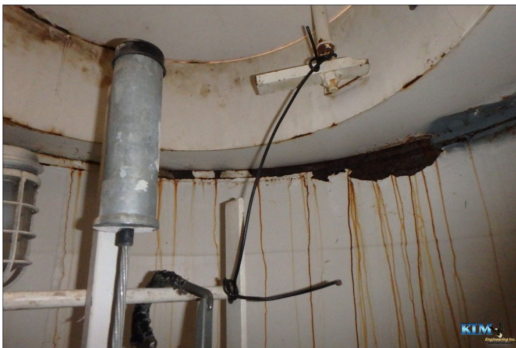
Photo No. 22 Condition of interior dry coating at top of drywell tube Significant peeling and surface corrosion occurring
