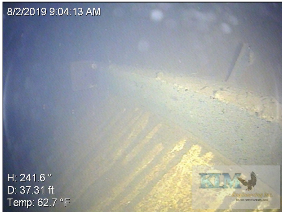
Photo No. 15 Condition of interior wet coating near tension ring Sediment accumulation and scale formation visible
