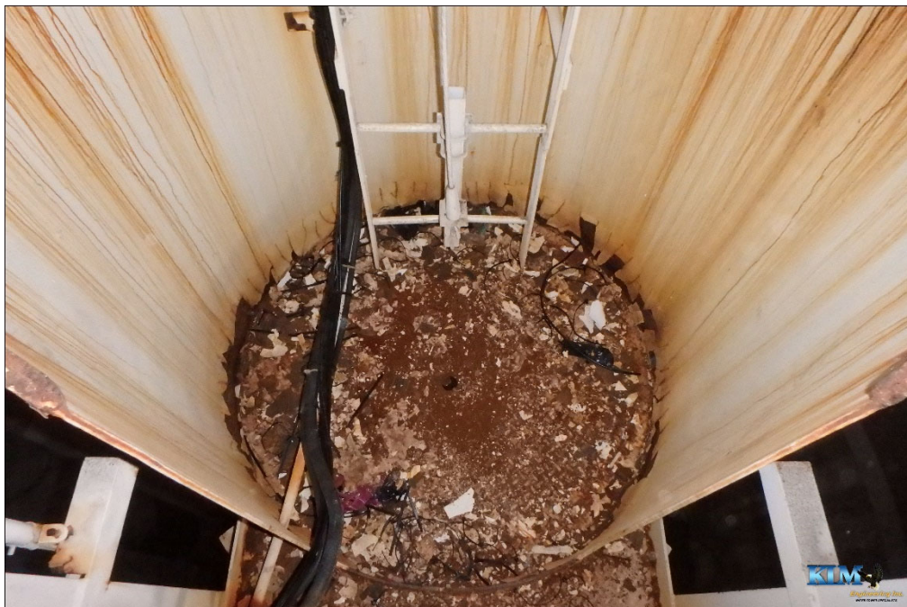
Photo No. 36 Condition of interior dry coating on drywell tube platform
