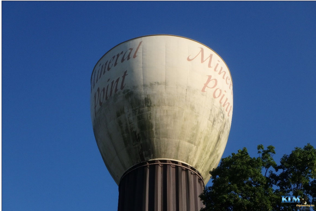
Photo No. 57 Overall condition of exterior coating on side of tank Heavy organic growth on lower half of tank
