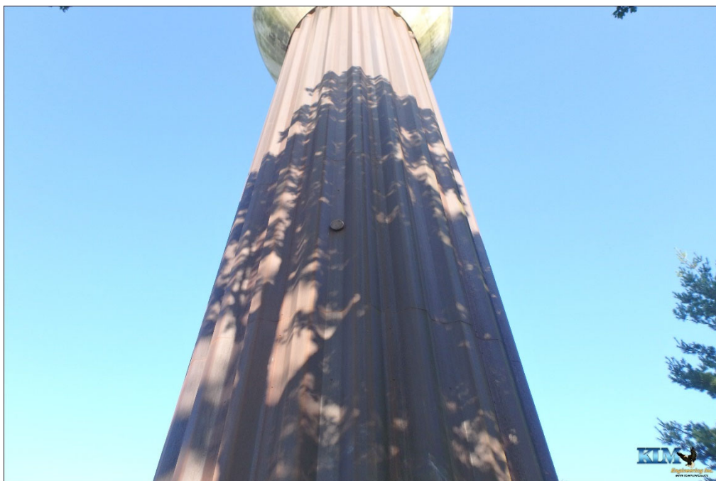
Photo No. 60 Condition of uncoated COR-TEN steel pedestal
