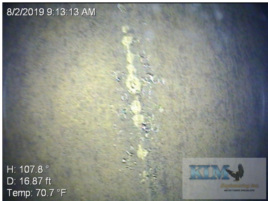
Photo No. 12 Condition of interior wet coating on shell wall Heavy scale and staining visible; coating blistering and pinhole corrosion along welds
