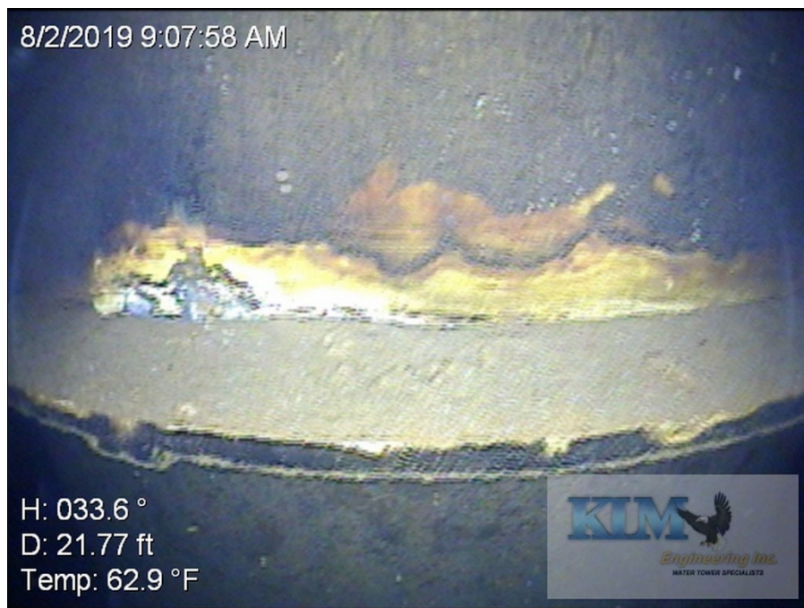
Photo No. 8 Condition of interior wet coating on drywell tube at stiffener ring Rust coloration due to corrosion
