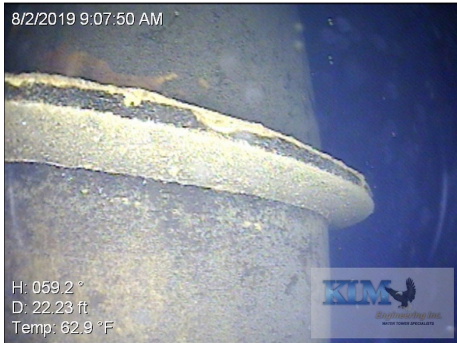
Photo No. 9 Condition of interior wet coating on drywell tube at a stiffener ring
