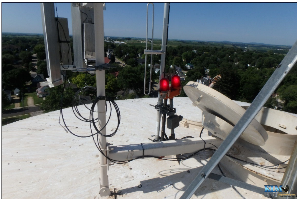
Photo No. 54 Condition of antenna mounts, drywell tube access hatch, and double aviation beacon
