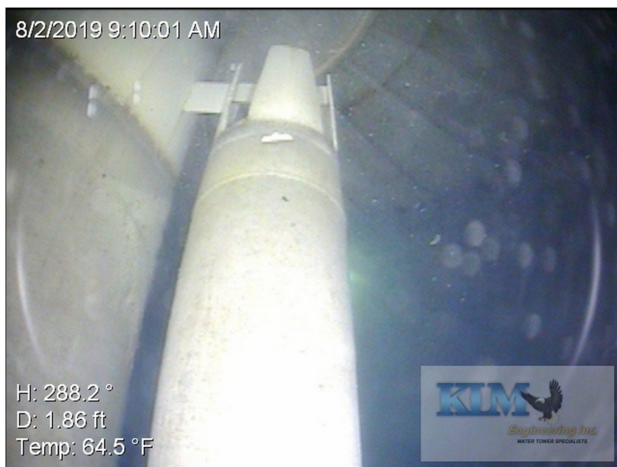
Photo No. 6 Condition of top of overflow pipe; view from below HWL
