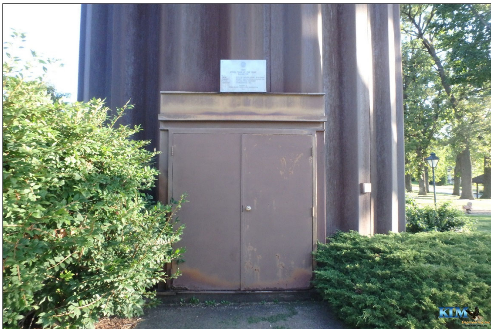
Photo No. 61 Condition of uncoated COR-TEN steel pedestal at base Double access doors significantly corroded at bottom corners
