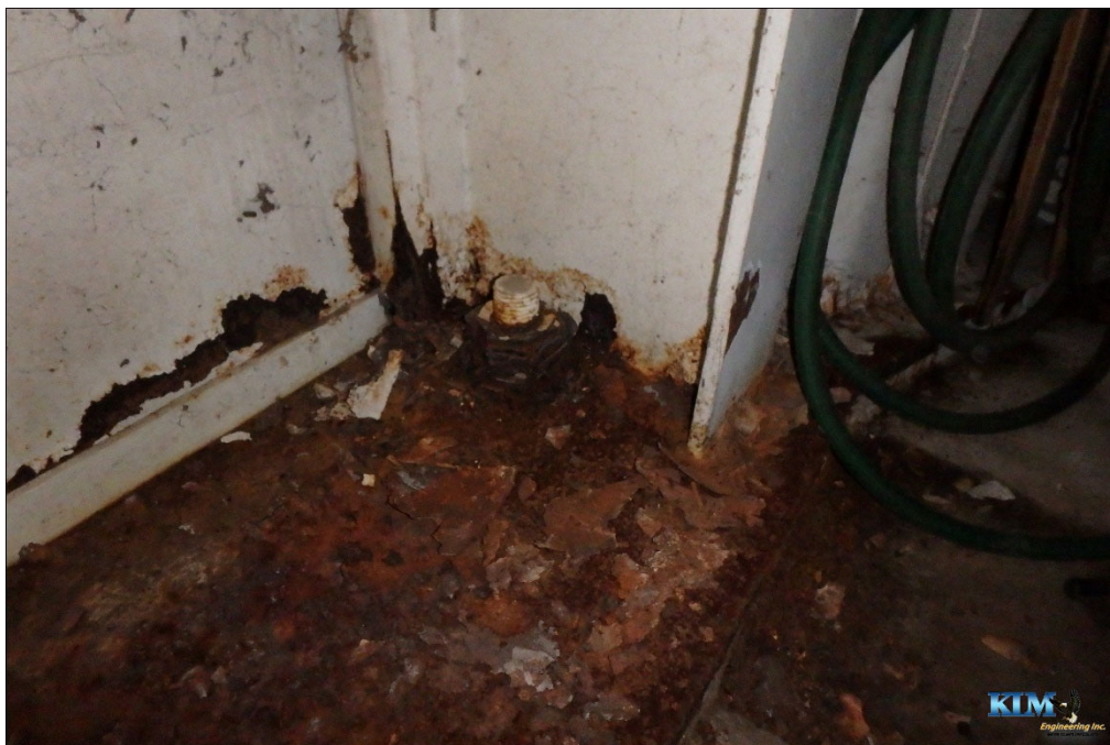
Photo No. 48 Condition of interior wet coating at base pedestal at double access doors Severe corrosion occurring on doors and on door frame
