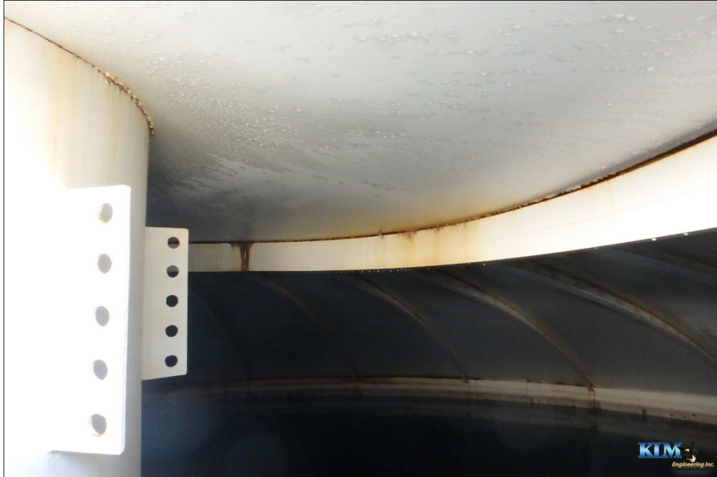
Photo No. 3 Condition of interior wet coating on roof around compression ring
