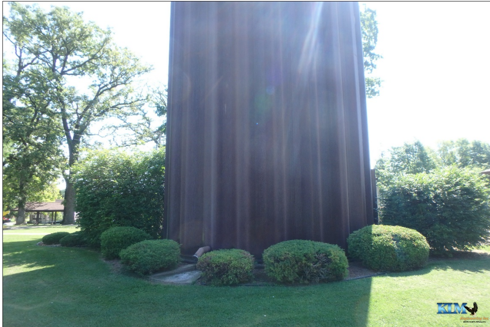
Photo No. 63 Site conditions around base of tower
