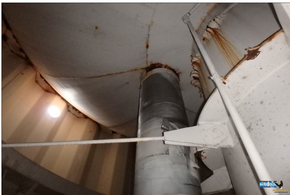
Photo No. 32 Condition of interior dry coating on bowl, drywell tube, fill pipe connection, and upper wall Random locations of heavy coating peeling and surface corrosion
