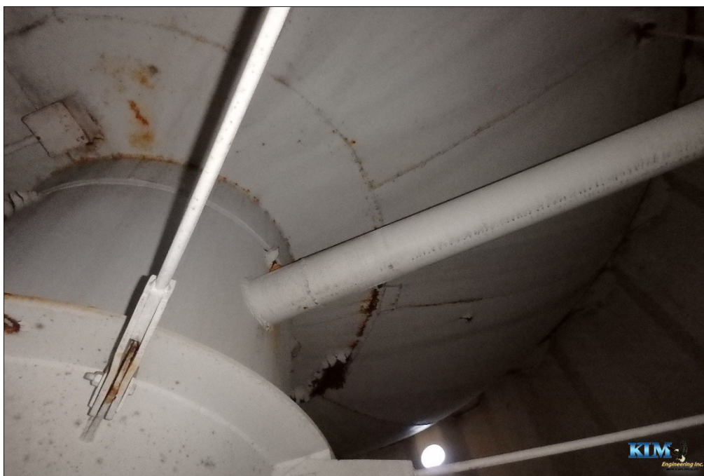
Photo No. 30 Condition of interior dry coating on bowl and drywell tube Random locations of heavy coating peeling and surface corrosion
