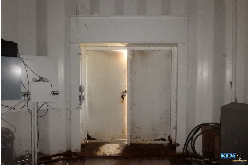
Photo No. 47 Condition of double access doors at base of pedestal Doors are severely corroded in bottom corners
