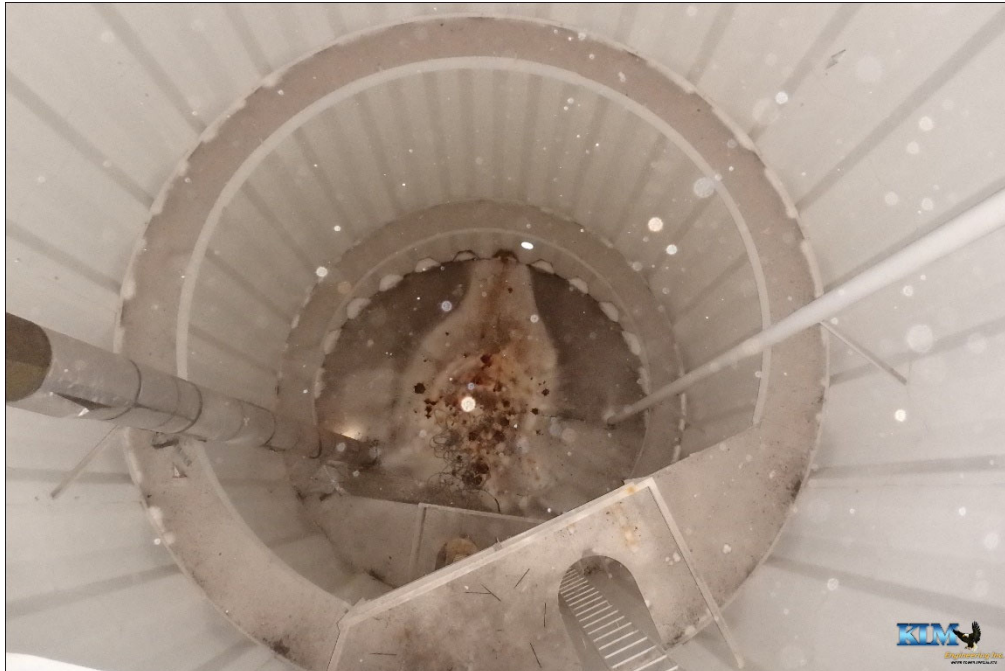
Photo No. 39 Condition of interior dry coating inside pedestal View looking down pedestal to condensate ceiling below
