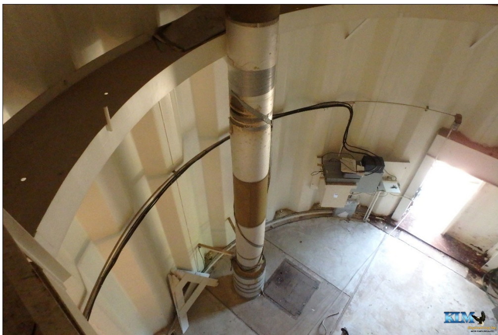
Photo No. 44 Condition of pedestal interior at base Some missing foil wrap visible
