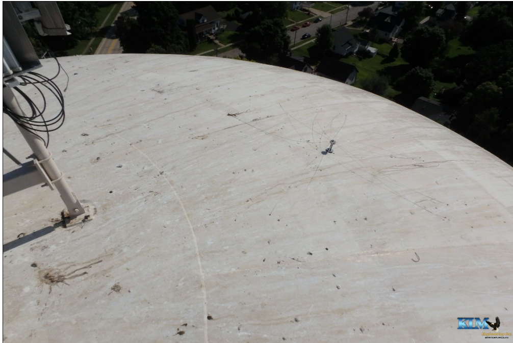
Photo No. 55 Condition of exterior coating on roof Bird droppings covering roof; non-functional bird deterrent visible
