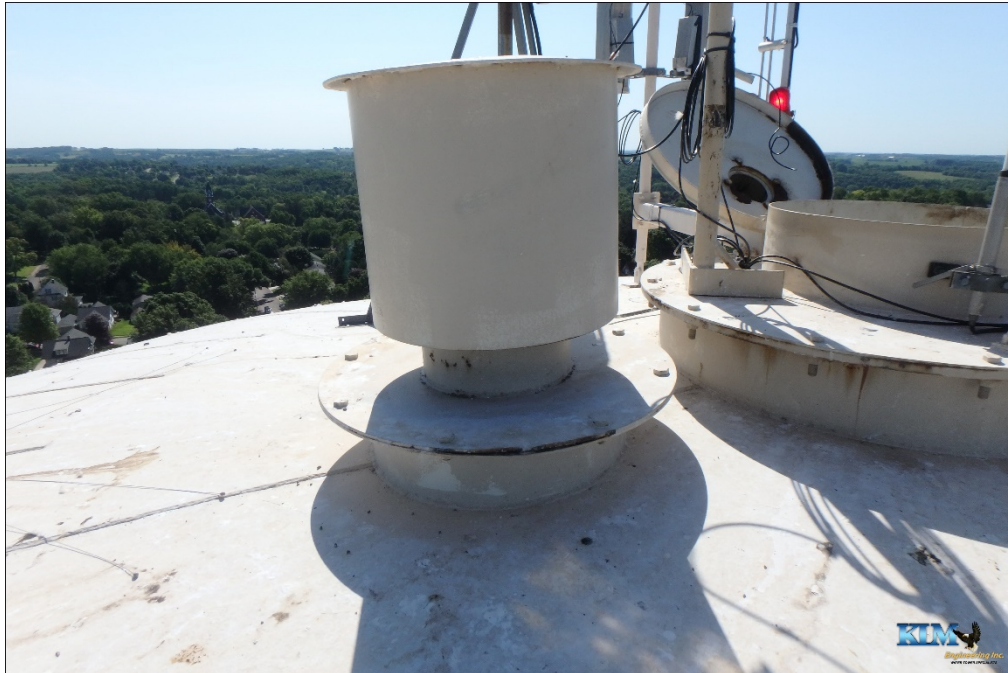
Photo No. 53 Condition of existing tank vent
