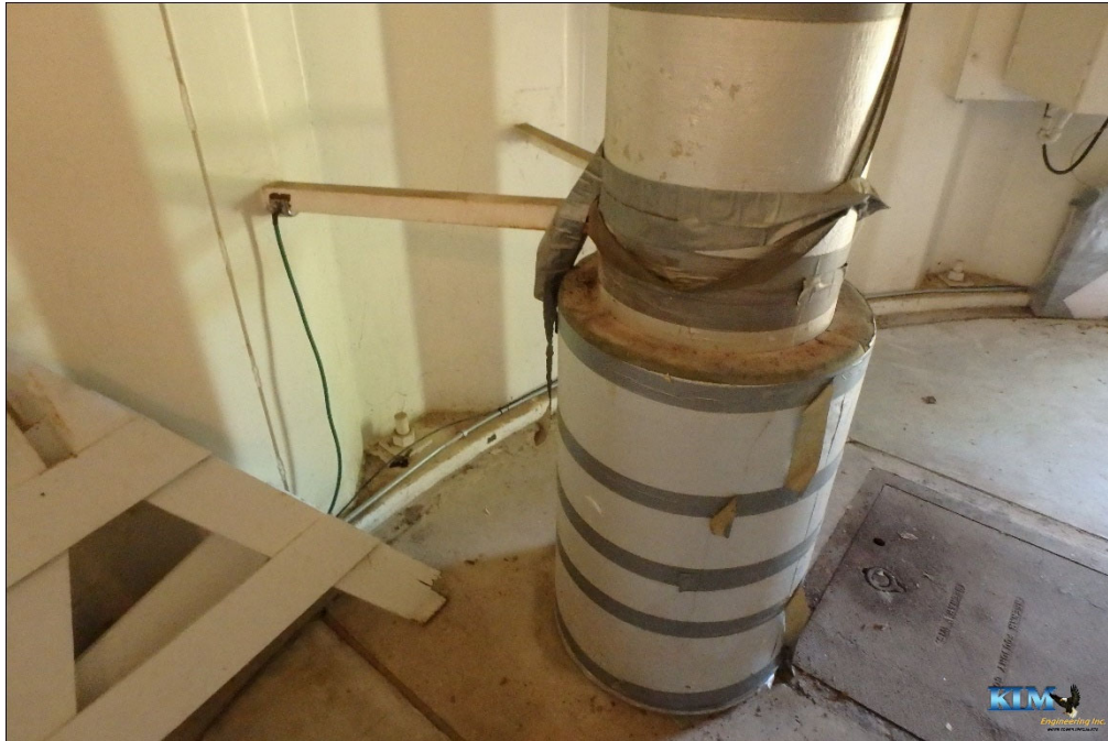
Photo No. 45 Condition of insulation and wrap on fill pipe at base of pedestal Hatch to valve pit visible
