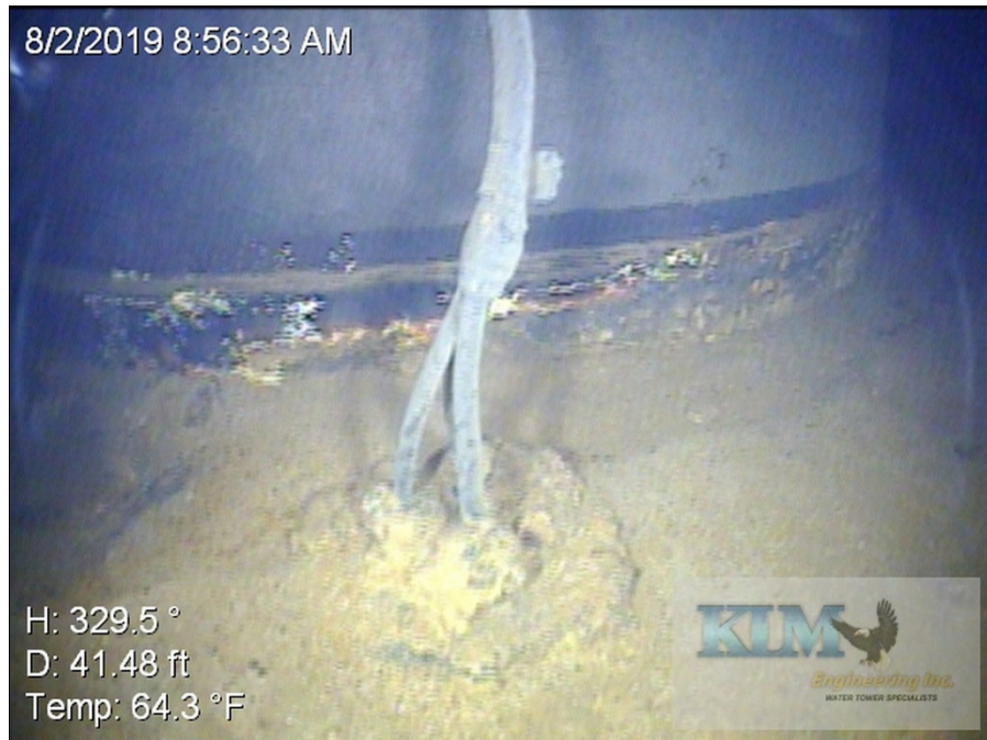
Photo No. 19 Condition of interior wet coating at base of drywell tube Cathodic protection cables visible
