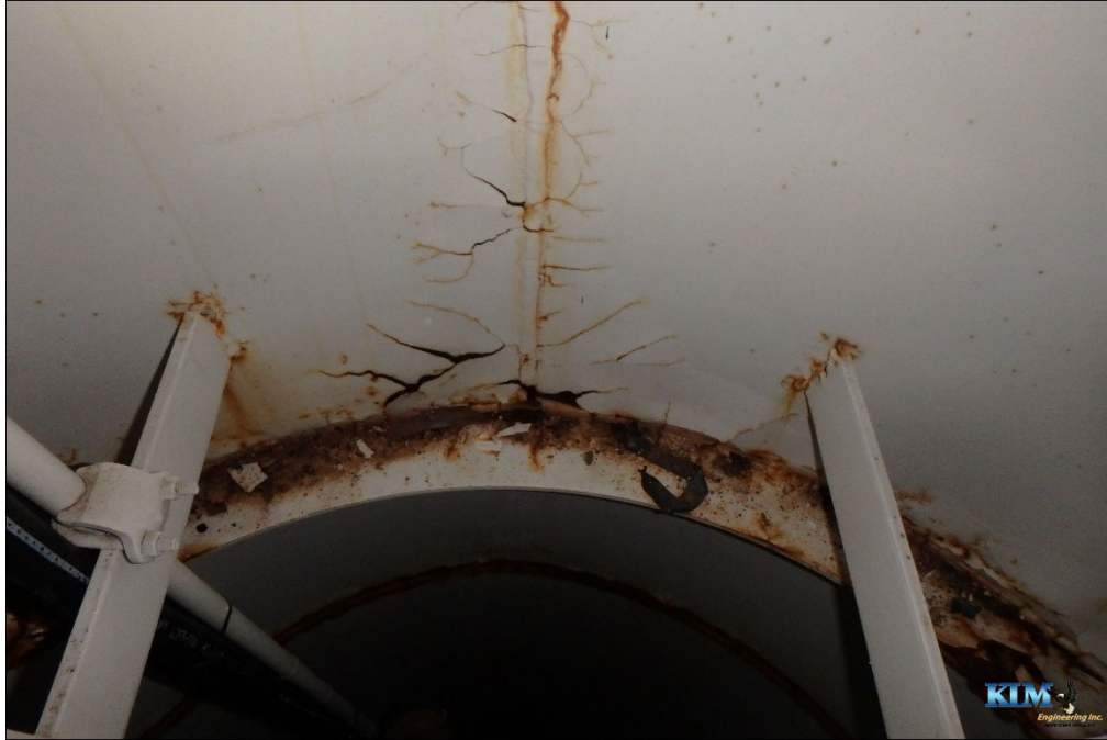
Photo No. 25 Condition of interior dry coating inside drywell tube Significant coating peeling and surface corrosion
