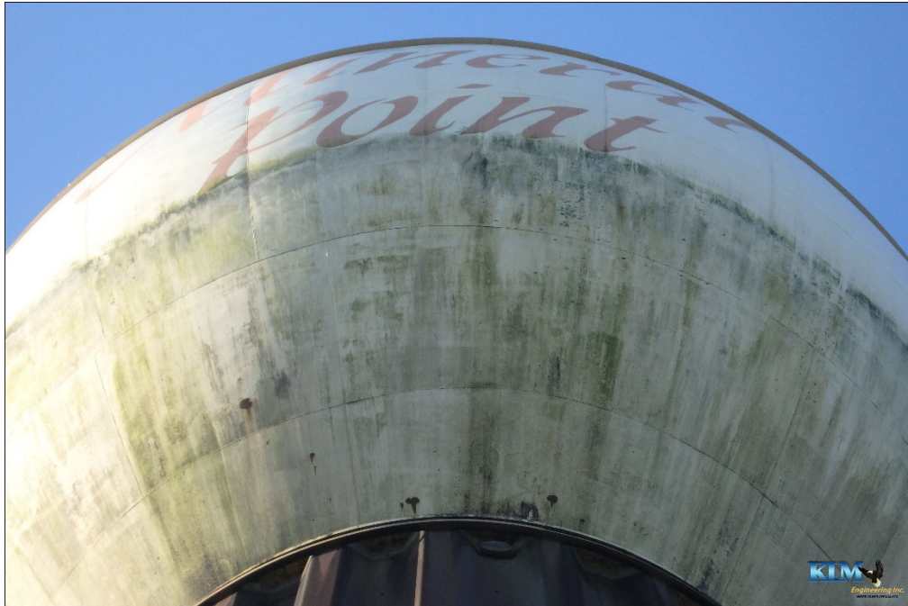
Photo No. 59 Condition of exterior coating near base of tank Spot and surface corrosion visible
