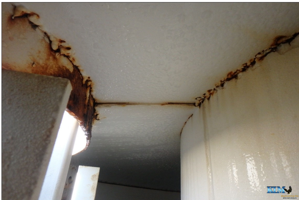
Photo No. 5 Condition of interior wet coating around drywell tube and manway access
