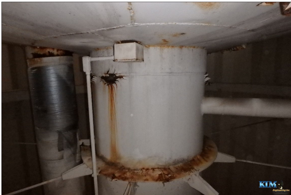
Photo No. 34 Condition of interior dry coating on drywell tube Cathodic protection system conduit and junction box visible
