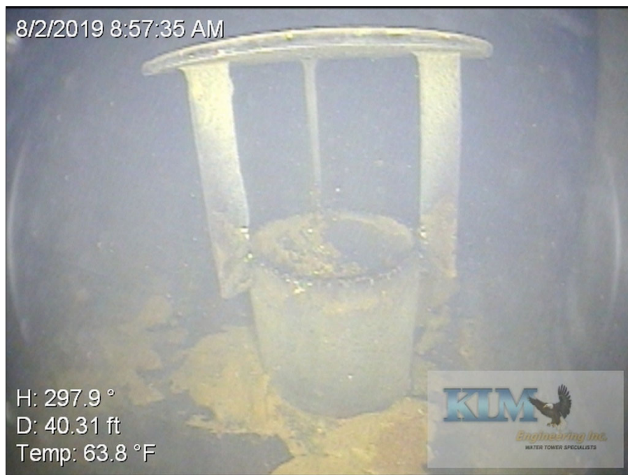
Photo No. 20 Condition of fill pipe in bowl Sediment accumulation visible around pipe
