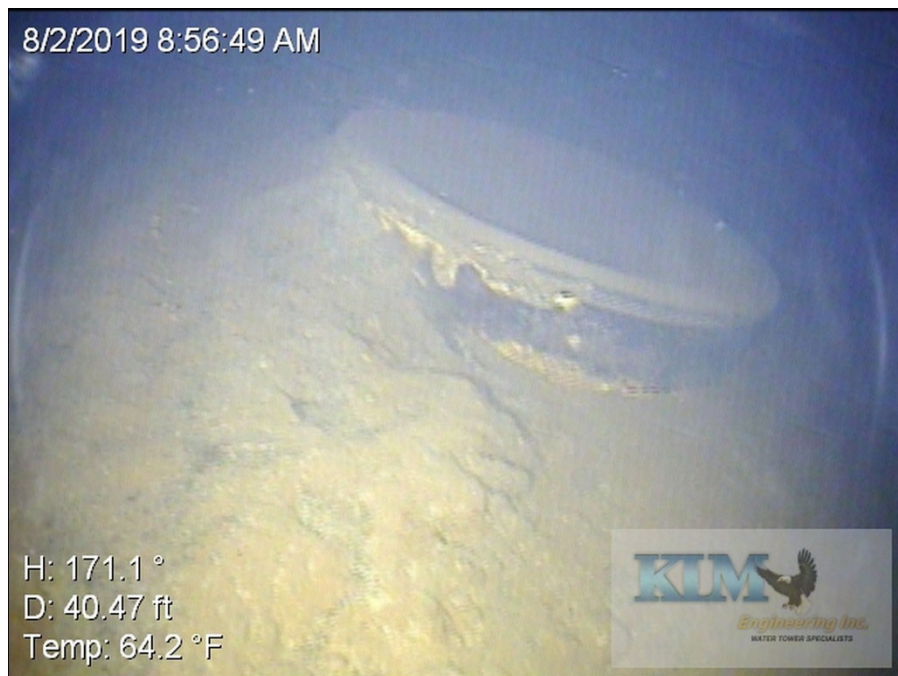
Photo No. 18 Heavy sediment accumulation and scale deposits in bowl Bowl manway visible
