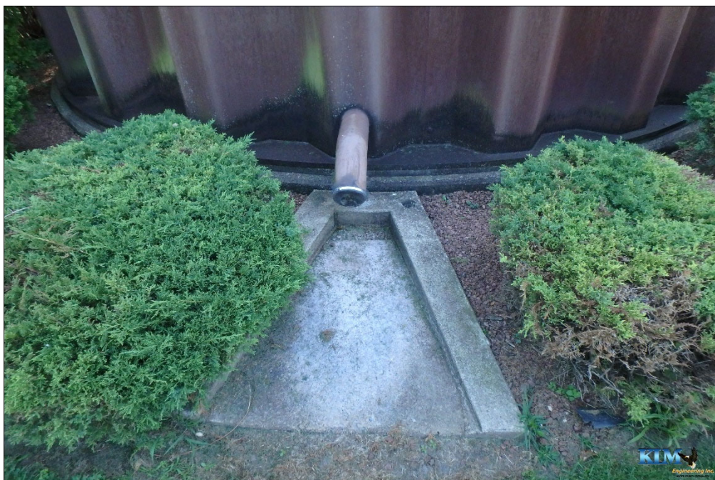
Photo No. 62 Condition of overflow pipe and splash pad at base of tower
