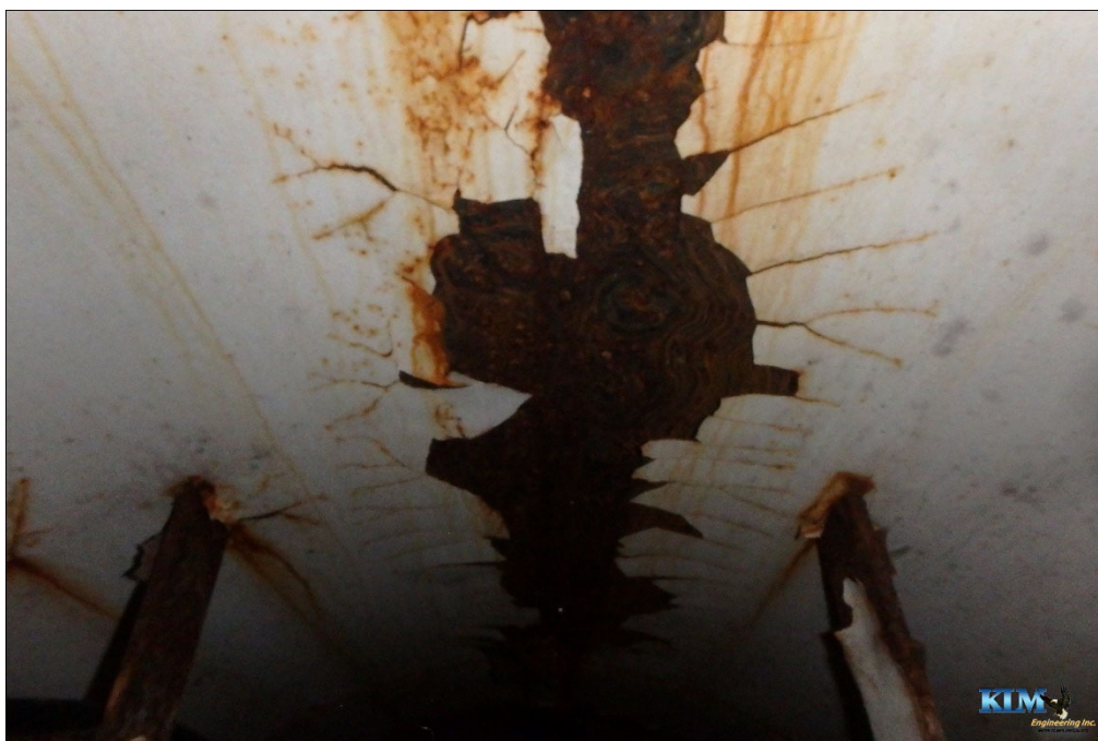
Photo No. 28 Condition of interior dry coating inside drywell tube Significant coating peeling and surface corrosion
