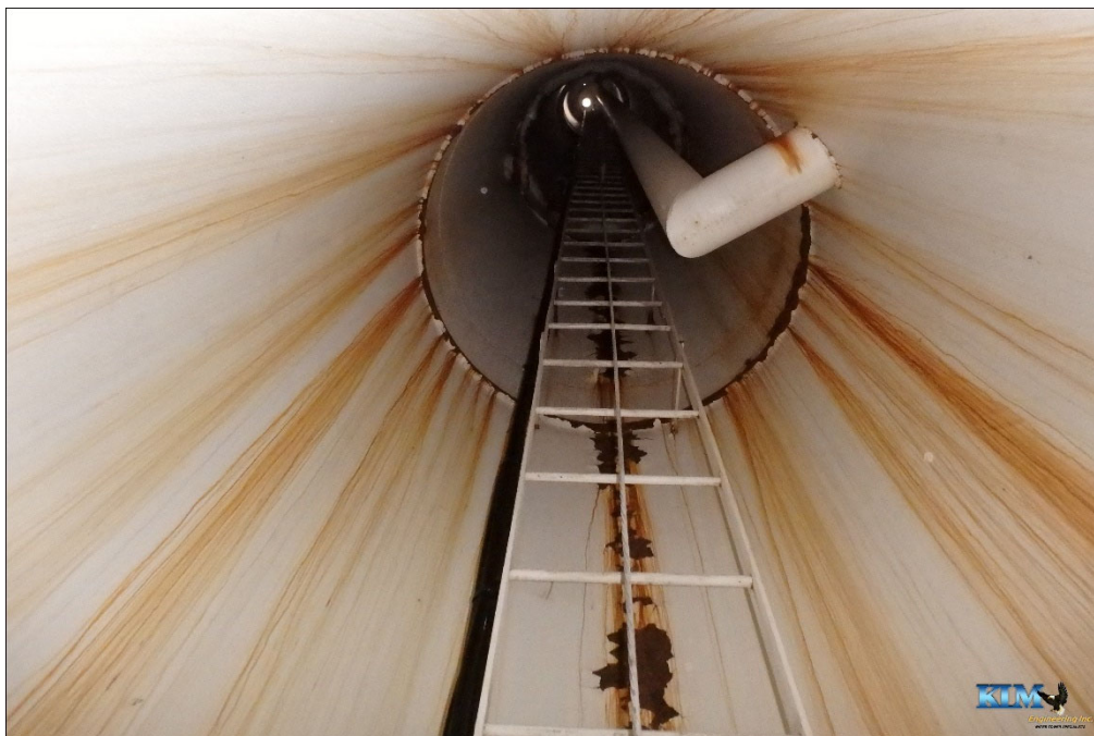
Photo No. 29 Condition of interior dry coating inside drywell tube Significant coating peeling and surface corrosion; staining from corrosion areas
