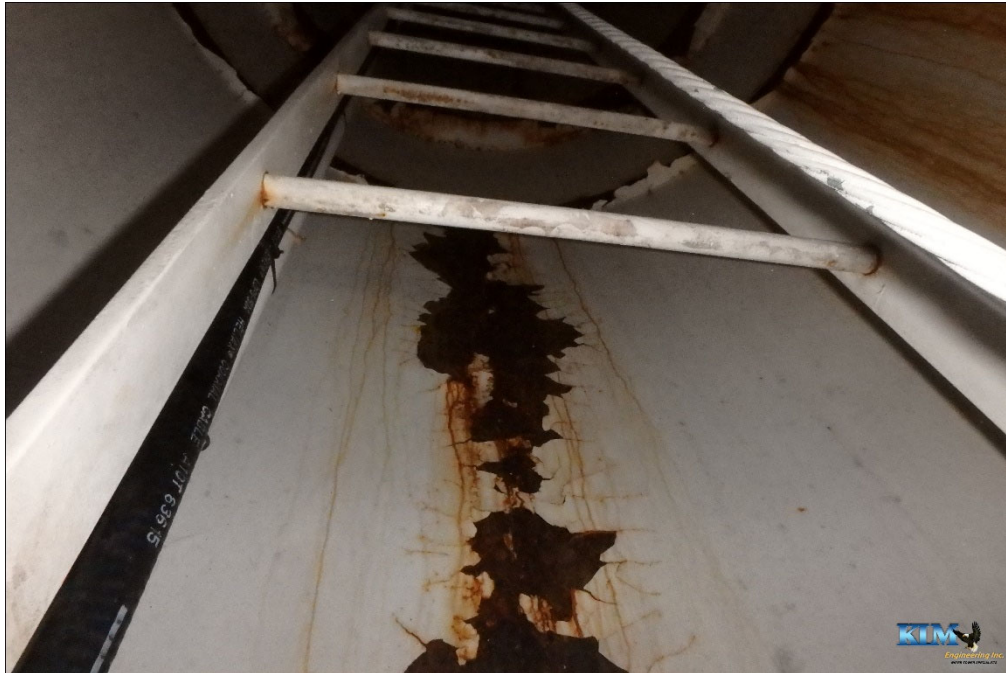
Photo No. 27 Condition of interior dry coating inside drywell tube Significant coating peeling and surface corrosion
