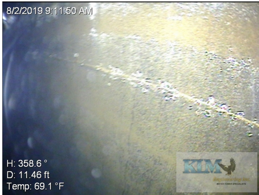
Photo No. 11 Condition of interior wet coating on shell wall Heavy scale and staining visible; coating blistering and pinhole corrosion along welds
