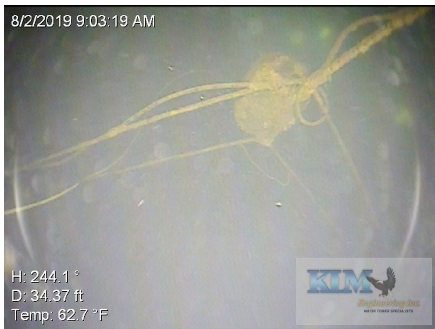
Photo No. 14 Submerged cathodic protection system
