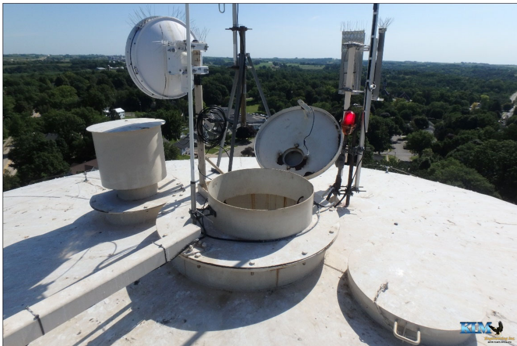
Photo No. 52 Overall view exterior roof condition
