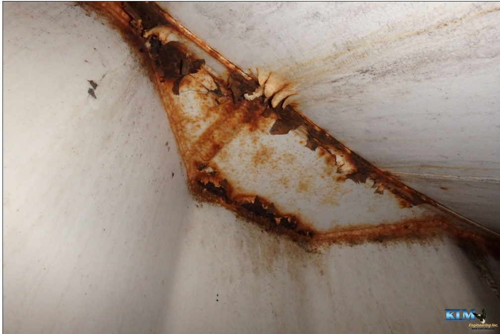
Photo No. 33 Condition of interior dry coating on bowl to wall connections
