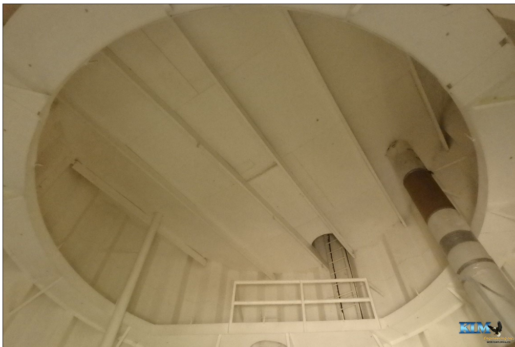
Photo No. 46 Condition of interior dry coating on bottom of condensate platform
